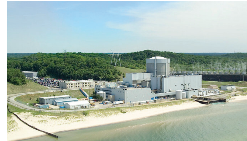
Palisades Nuclear Generating Station
